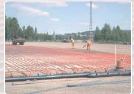
Installation of Uponor Surface Heating System
