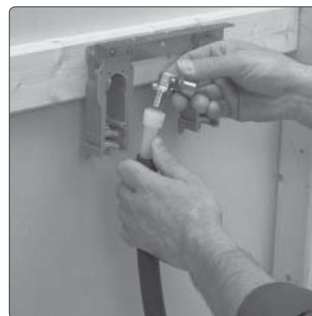
3. Montera Q&E-koppling.
