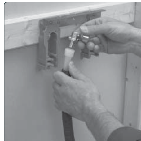
3. Montera Q&E-koppling.
